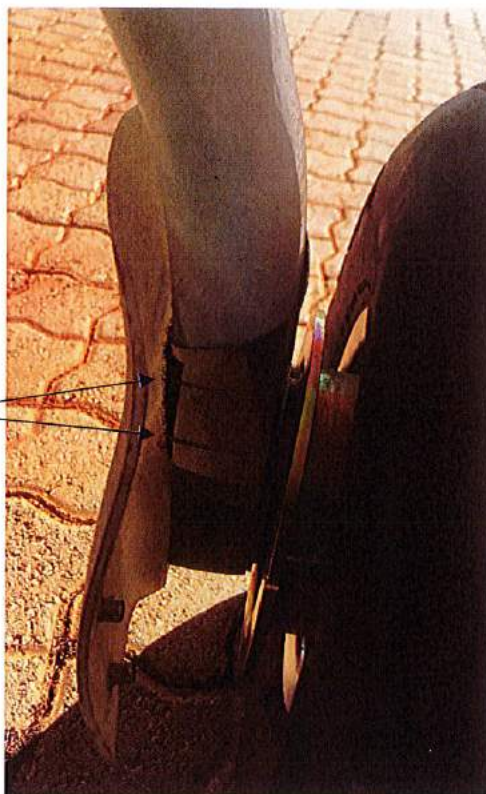
Figure 3 – Installed heat shield
