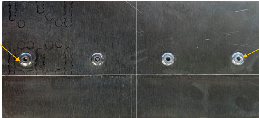
Figure 4 – Identification of stainless steel and aluminium rivets
