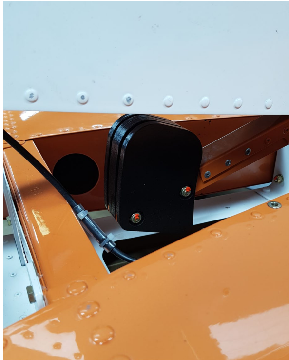
Figure 1 Elevator centre balance weight visible after removing empennage fairing
